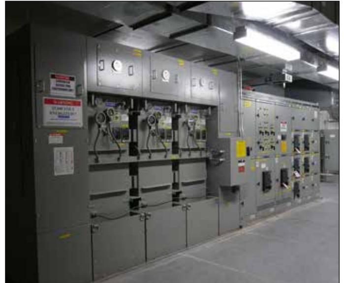
Figure 15. Triplex Indoor Power Center comprising of energy efficient and low noise single-phase substation transformers in a ganged setup.
